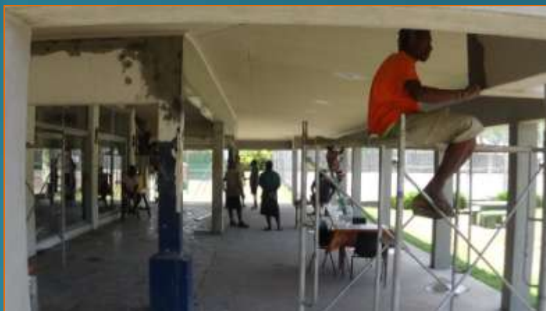
New terrace and ceiling, October
