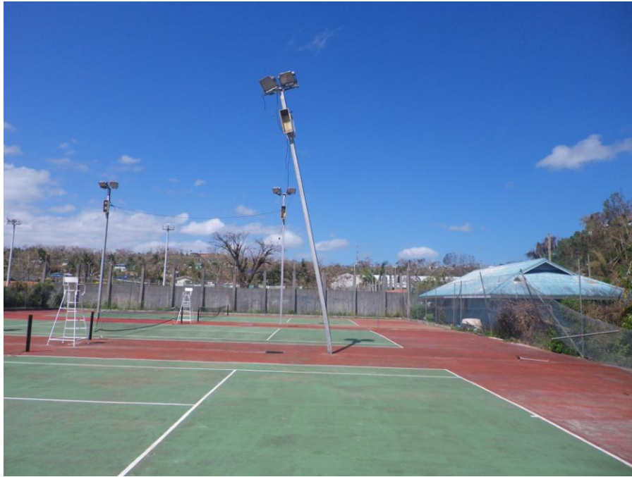
Light posts bent by wind
